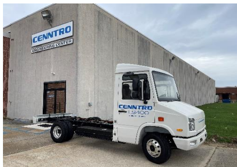
New Jersey Assembly Facility
